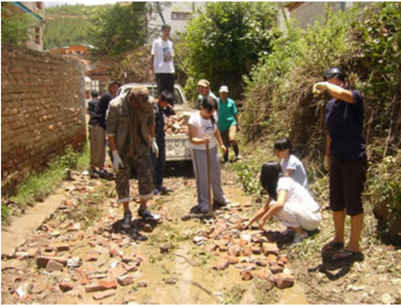
Filling the road, creating a footpath for the pedestrians.
